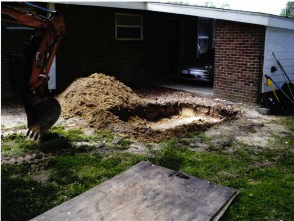
Picture 2: UST 1271Dove excavation in progress.
