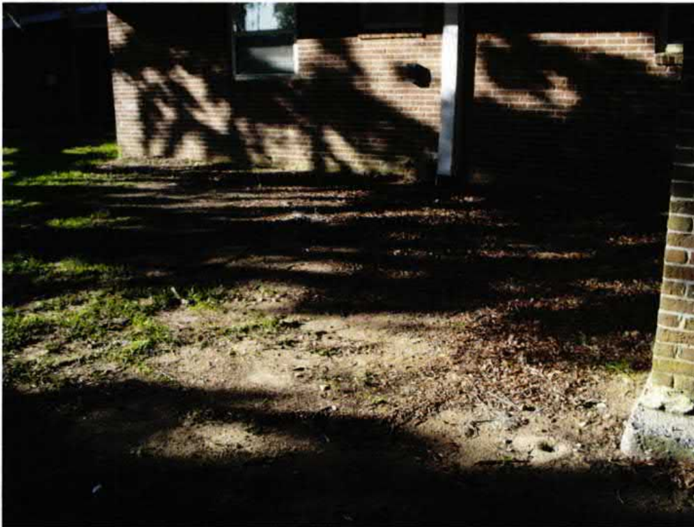
Picture 1: Location of UST 1271Dove.
